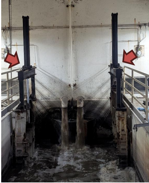
Existing Headworks Influent Gates
