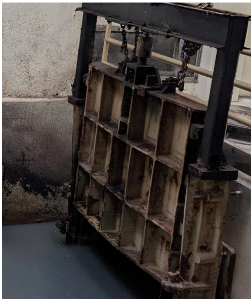
Existing Cast-Iron Sluice Gate
