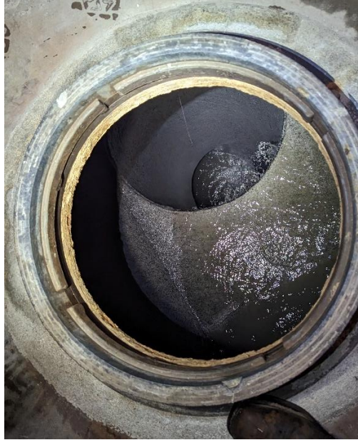
Manhole on influent deck to be used for Flow Bypass System
